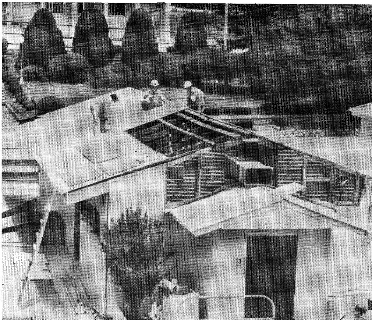
ICC workmen replace the roof on Building T-3. The original framework was left intact.
